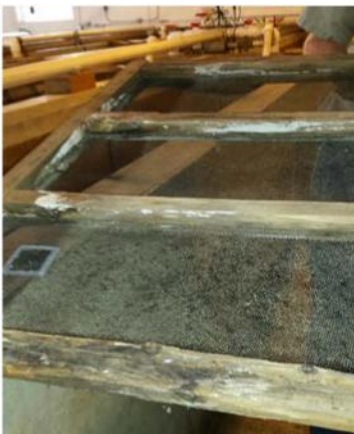
Figure 11: Rotting fish screen, one of several maintenance issues observed at ODFW hatcheries
